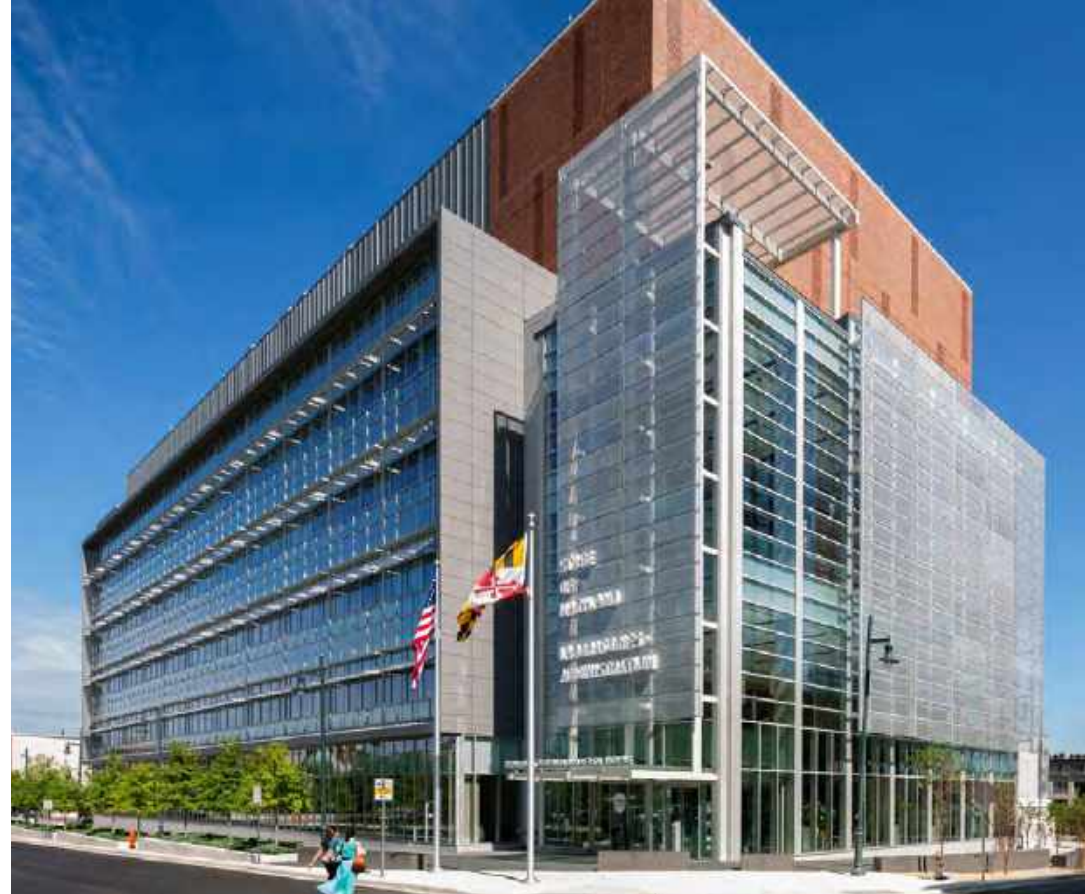
EXAMPLES: ARTICULATED CORNERS IN MODERN OR TRADITIONAL STYLES TOP: BIO-INNOVATION CENTER, NEW ORLEANS BELOW: MIXED-USE BUILDING, ANNAPOLIS TOWN CENTER
